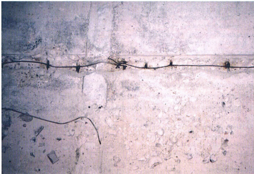
Figure 7: Establishing electrical continuity between the reinforcing bars.
