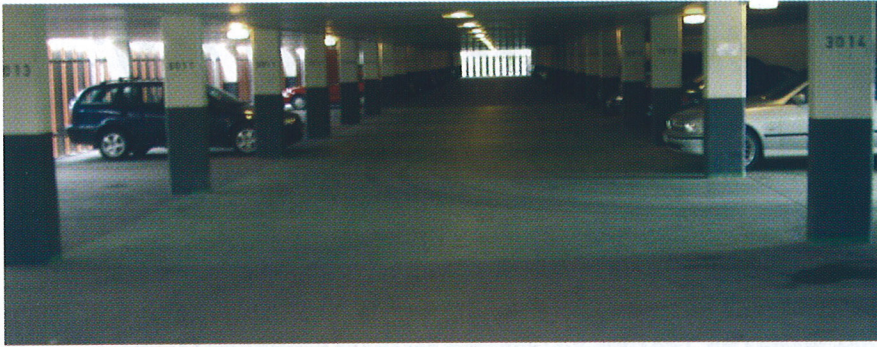
Figure 10: The car park after application of the water-resisting layer.
